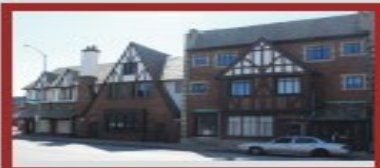
MANCHESTER APTS Transitional Housing 960 N. Pennsylvania St.
